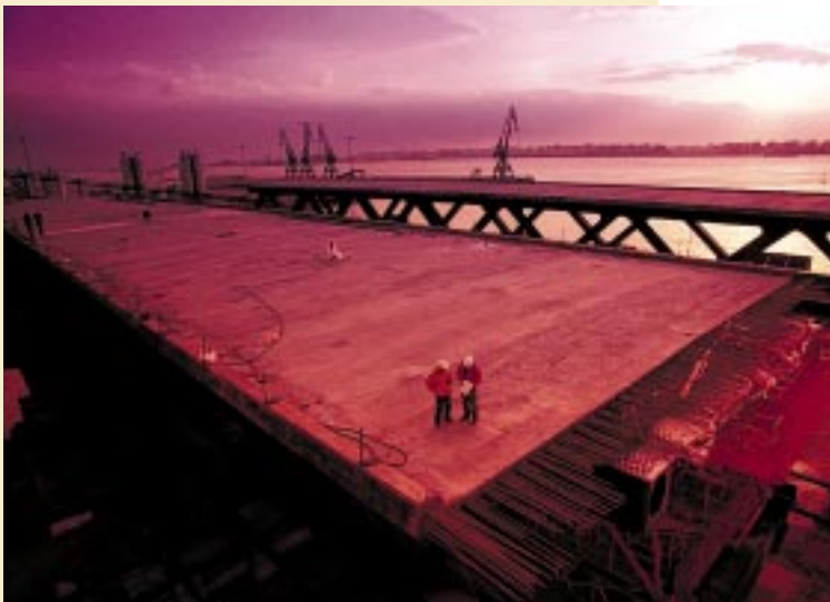
Building into the next millennium European bridge construction
