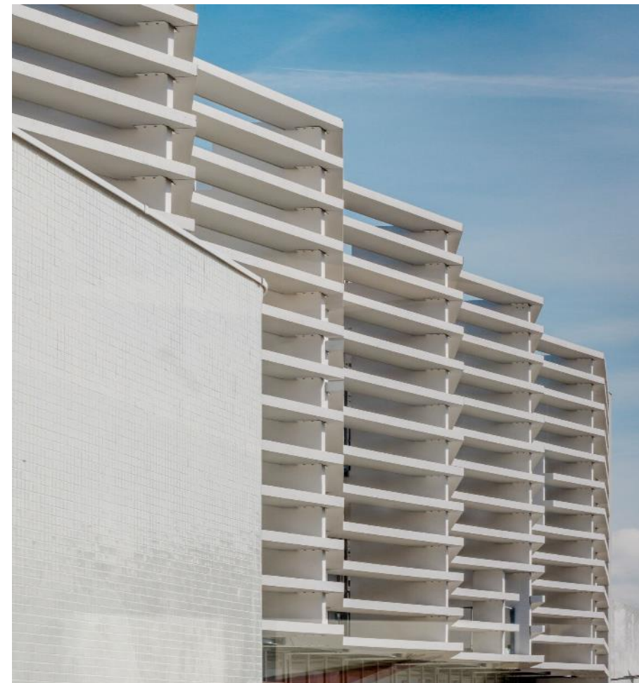
College Gilbert Charbroux, Lyon, France Built with Insularis, part of our Vertua family of sustainable products
