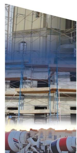
CEMEX Shotcrete concrete is a specially designed concrete developed for use with compressed air spraying equipment. Shotcrete is a fast and effective way to apply a concrete in areas where using conventional concrete would be difficult. CEMEX Shotcrete also forms an integral part of an innovative low cost, low carbon housing solution
