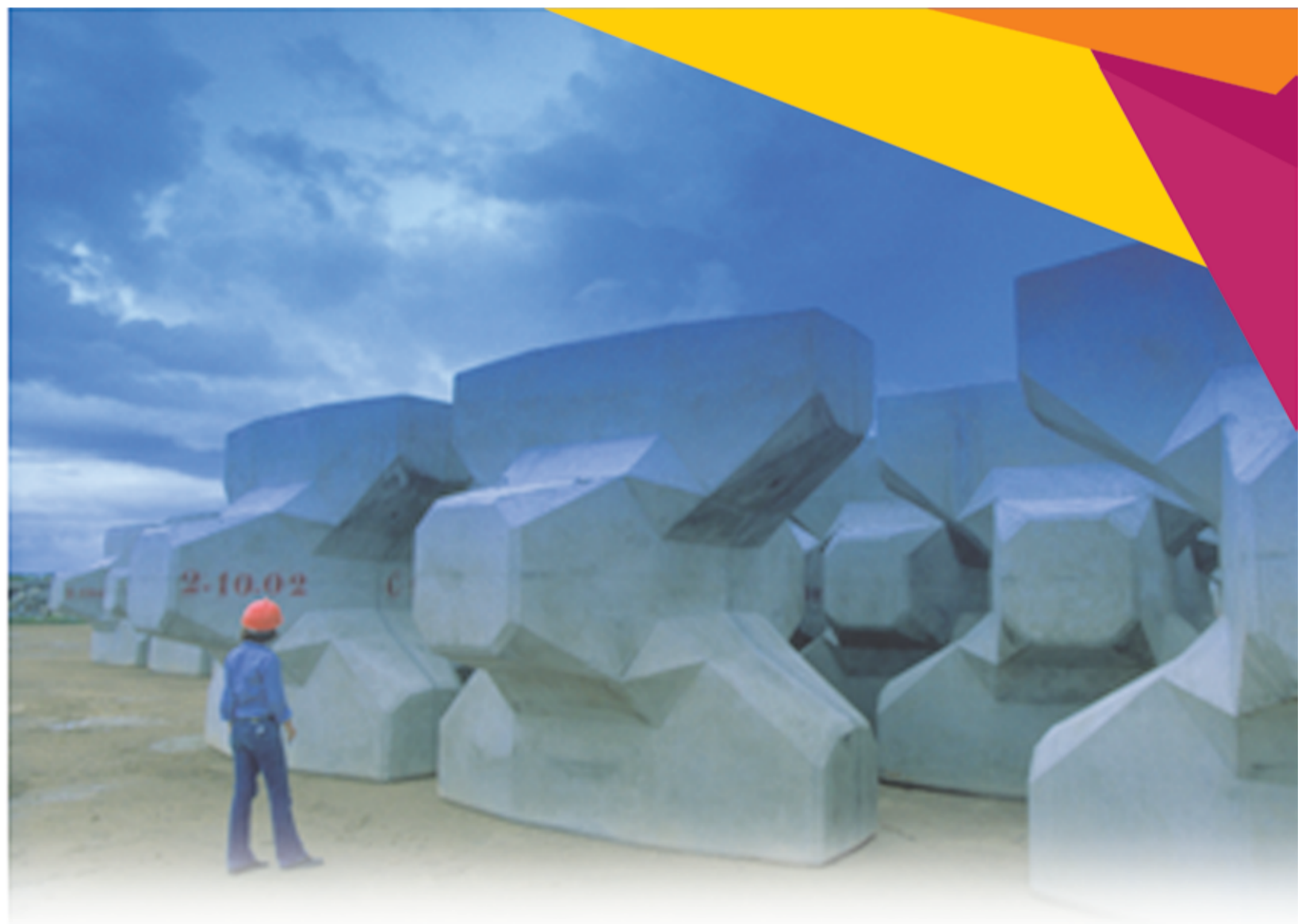
Precast concrete sea defenses in the Dominican Republic, made with CEMEX cement and expertise.
